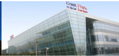
“East Park Trade Center” office building | Sofia (Bulgaria)
