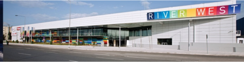
River West shopping center | Athens (Greece)
