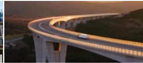
KRINKAL BRIDGE - SLOVENIA
